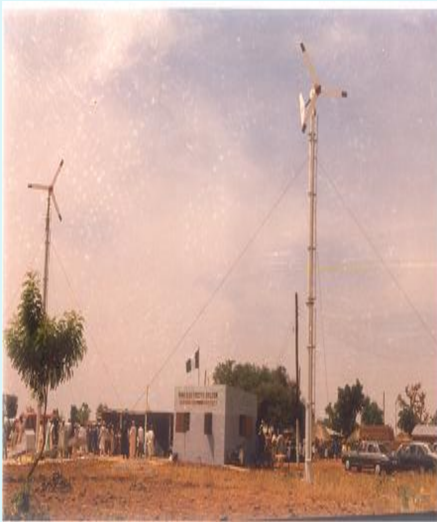
5kW aero generator in Sayya Gidan Gada, Sokoto State
